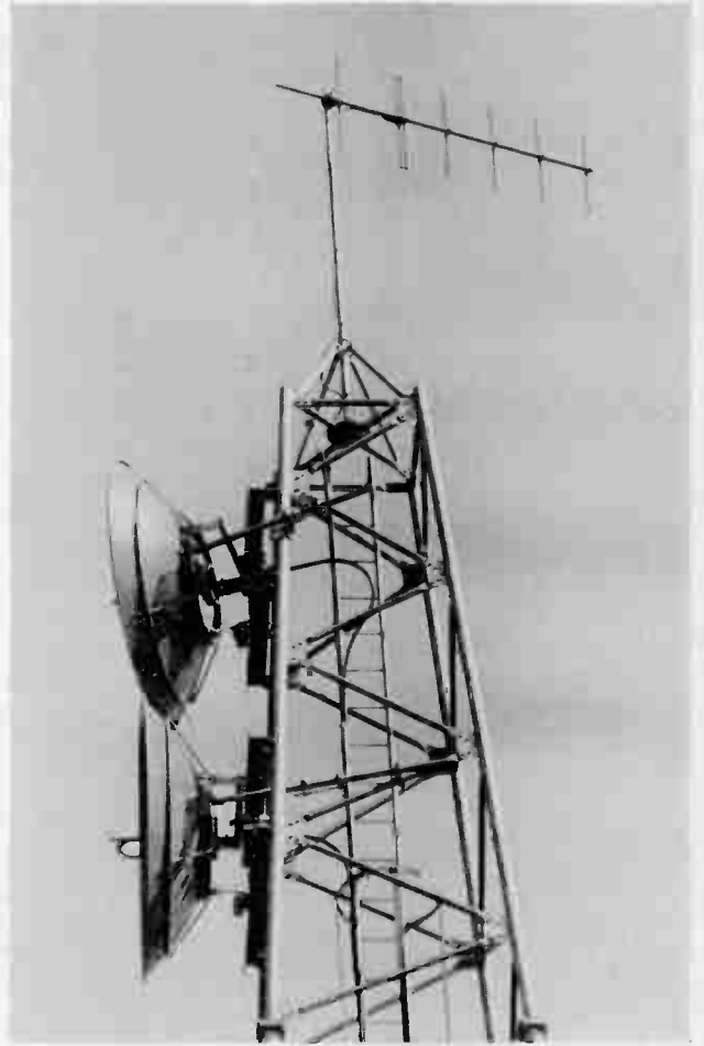
(c) 7000 MHz receiving aerials at Gravesend, for radar data signals from Broadness and Crayfordness.
