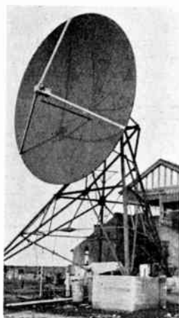
Fig. 5. 30 ft parabolic dish aerial with dual polarization horn feed.
