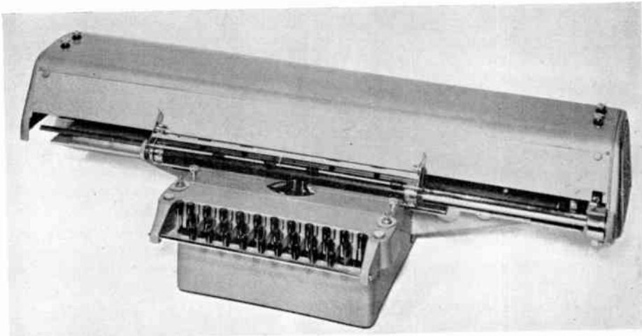
Fig. 9. Compuprinter mechanism—20 characters per second.
