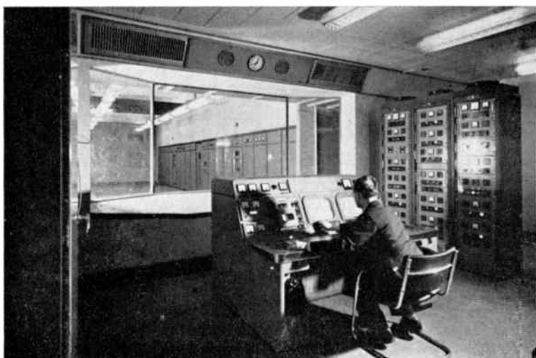
Fig. 4.—The Control Room, with a view of one bay of transmitters beyond, showing the control desk and the three racks containing the drive and phasing equipment.
