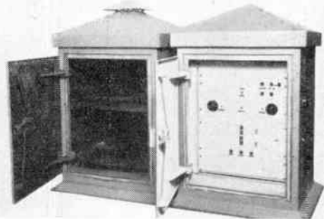
Fig. 13.—Unattended, single-programme, Rediffusion equipment housed in weatherproof kiosks.
