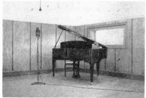
Fig. 19.—Corner of studio showing use of resonant panels.
