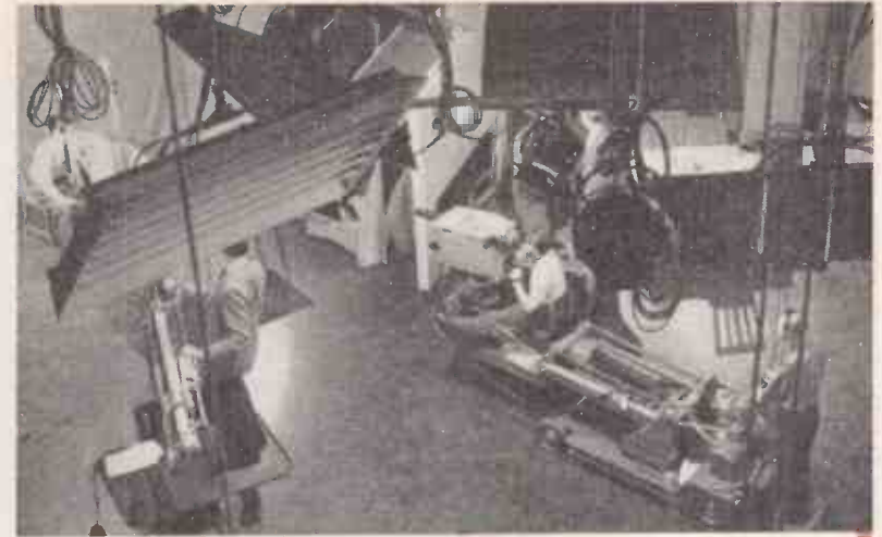
Associated-Rediffusion's New Wembley Television Studio Centre Studio 1. A view of Studio 1 from the lighting control position showing a Marconi television camera on the studio floor and the "bath tub" fluorescent lighting equipment with telescopic suspension from the lighting grid.
