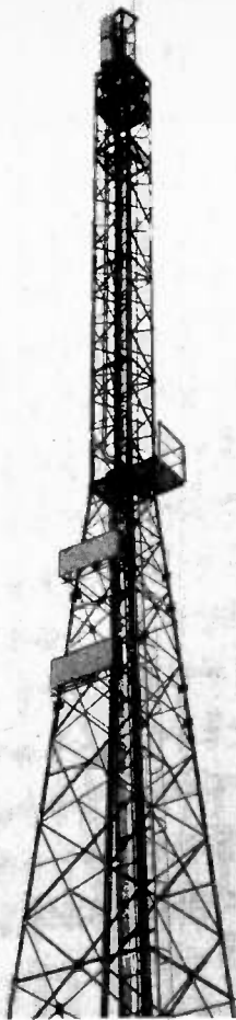
Cop Hill transmitting mast - an IBA relay transmitter of 1 kw erp
