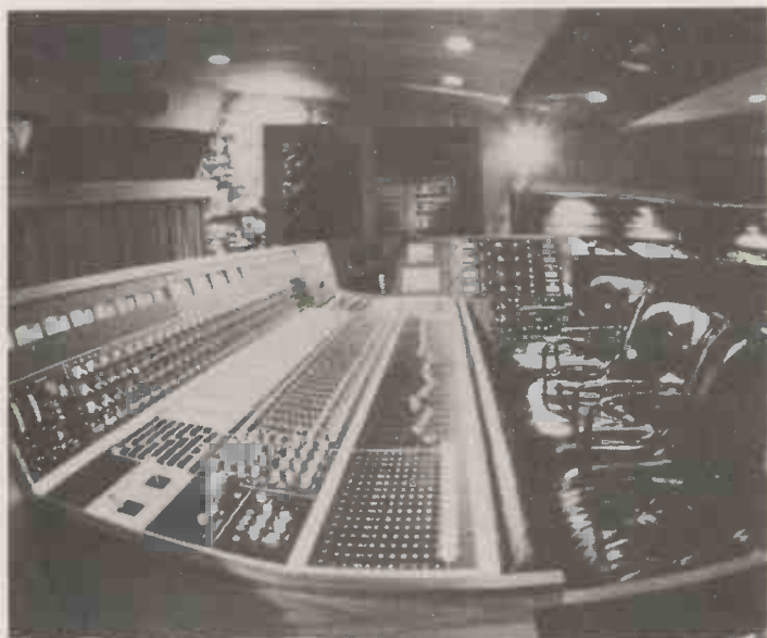
A fish-eye view of the control room at Threshold.
