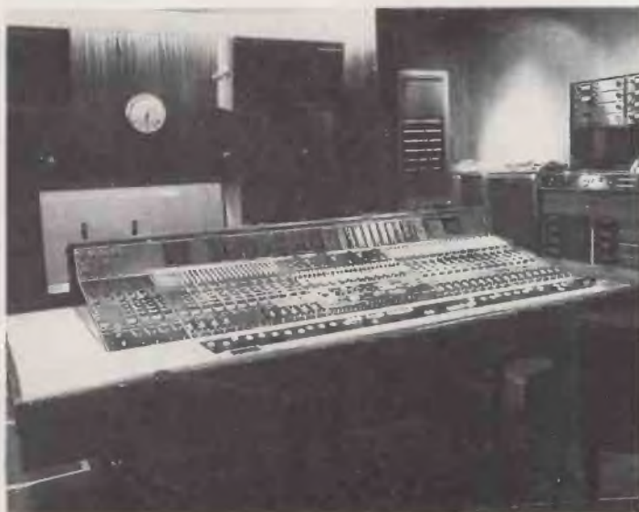
The main control room. The design of the Neve desk is important
