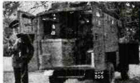
ABOVE: A BBC recording truck as used in Italy and elsewhere by BBC war correspondents. Observer J. R. N. Nixon and (in the truck) Recording Engineer G. P. Wade are operating the recording equipment, which includes two hundred yards of microphone cable.
