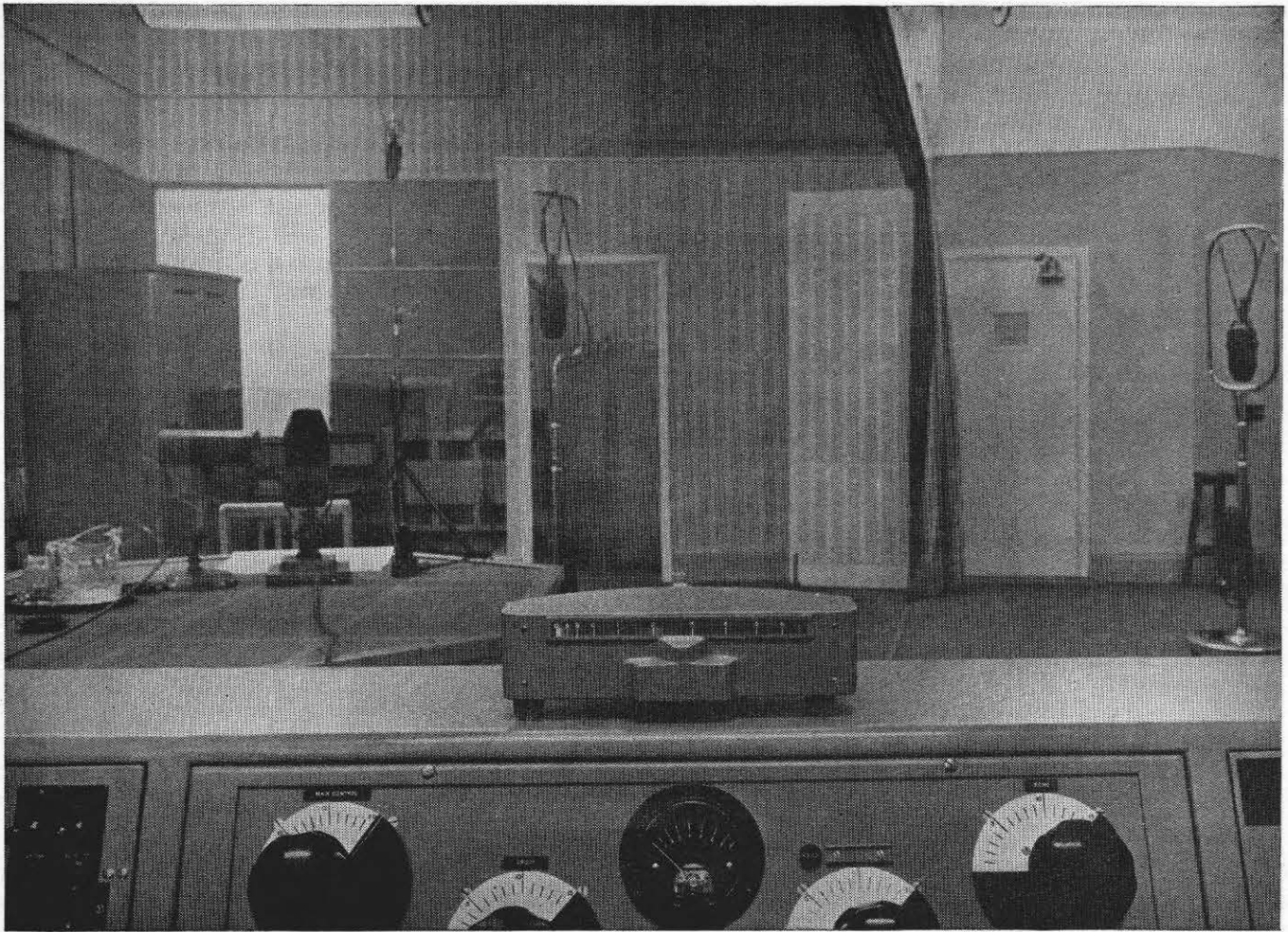
Fig. 6 — Installation in Drama Studio
