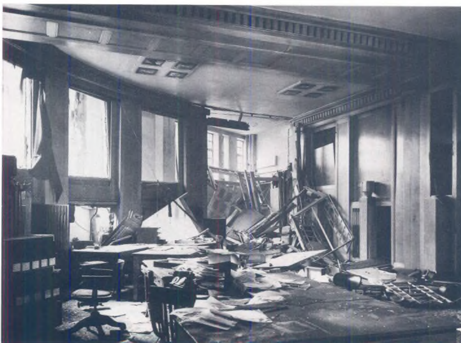
1940: Bomb damage in the Council Chamber
