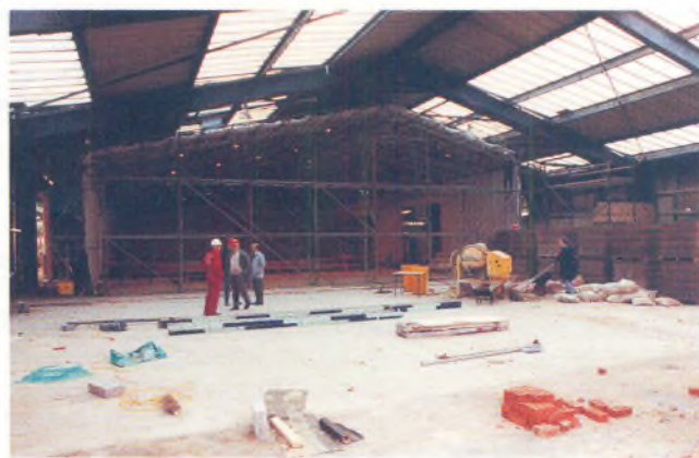
Stage One during construction (March 1991)
