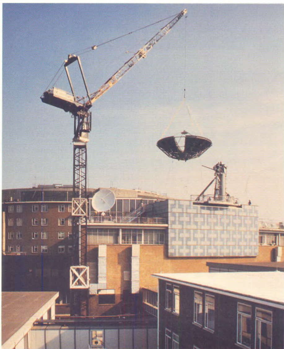
The 9 metre dish being hoisted onto the roof of Television Centre on 21st September
