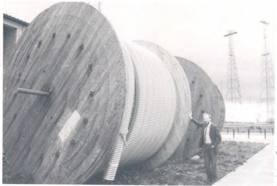
Skelton C: Peter Lamb dwarfed by the coaxial feeder awaiting installation
