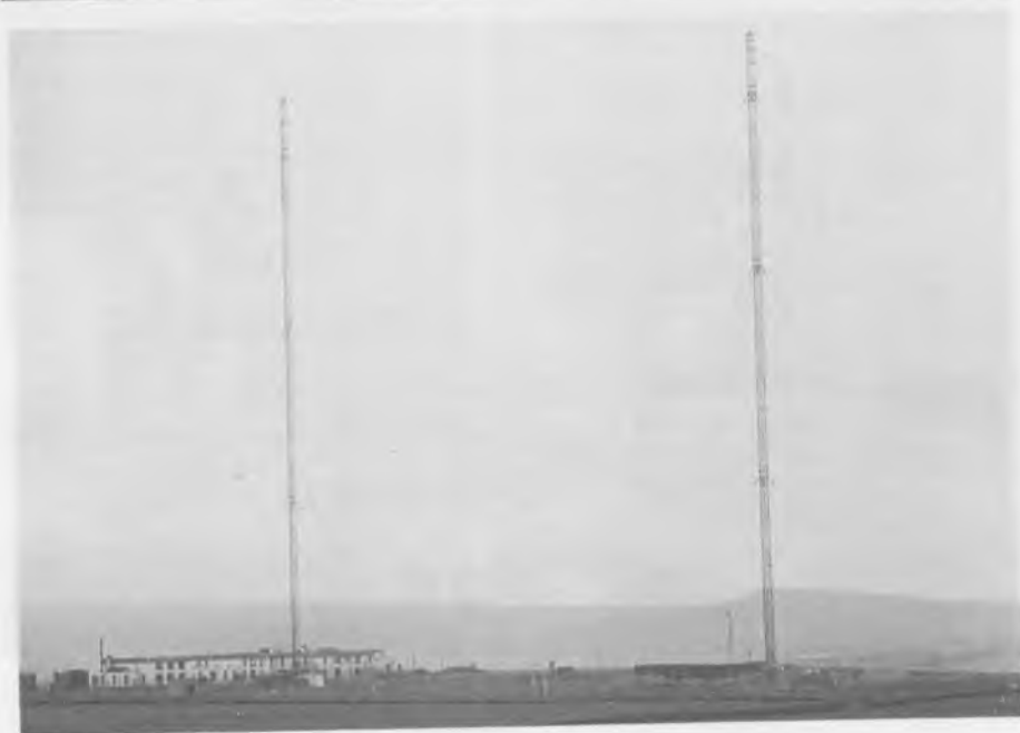
The old and new masts at Moorside Edge
