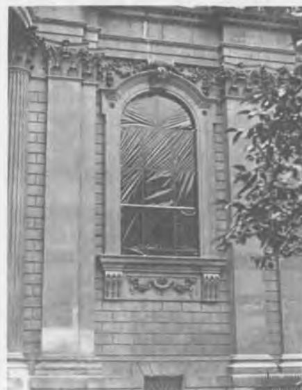
The orange plastic filter stretched over one of the Cathedral windows
