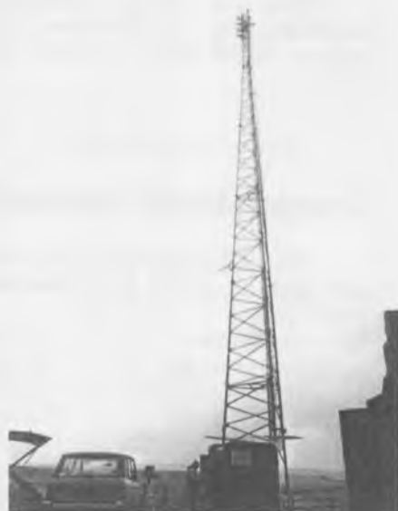
The Hedleyhope mast and transmitter cubicle being filmed as a possible TV news story
