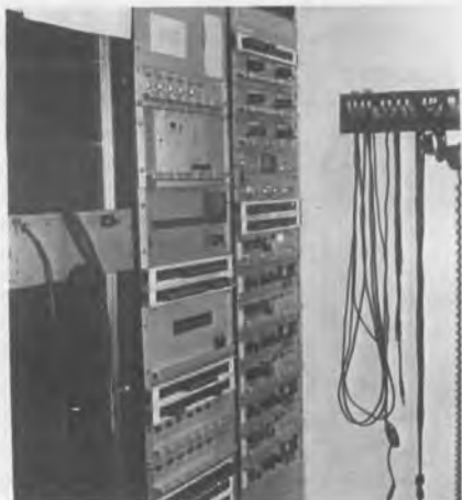
The new microprocessor control equipment under installation
