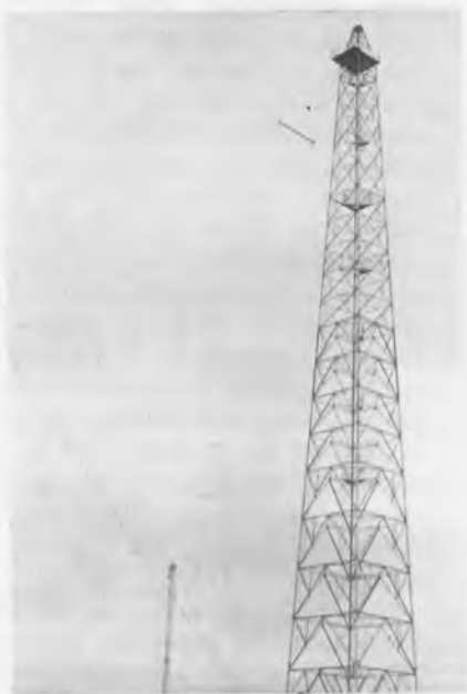
A multi-band HF aerial array
