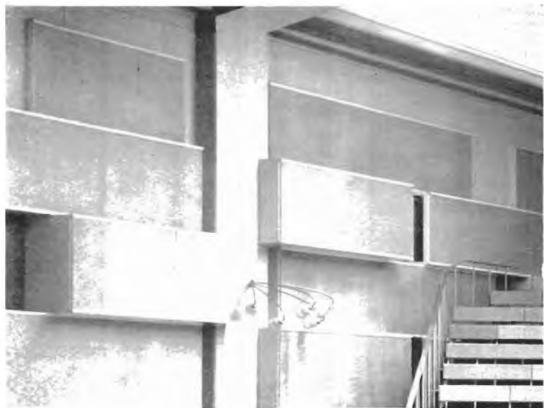
Plate 3.1. Part of Studio 1, Maida Vale, showing membrane absorbers
