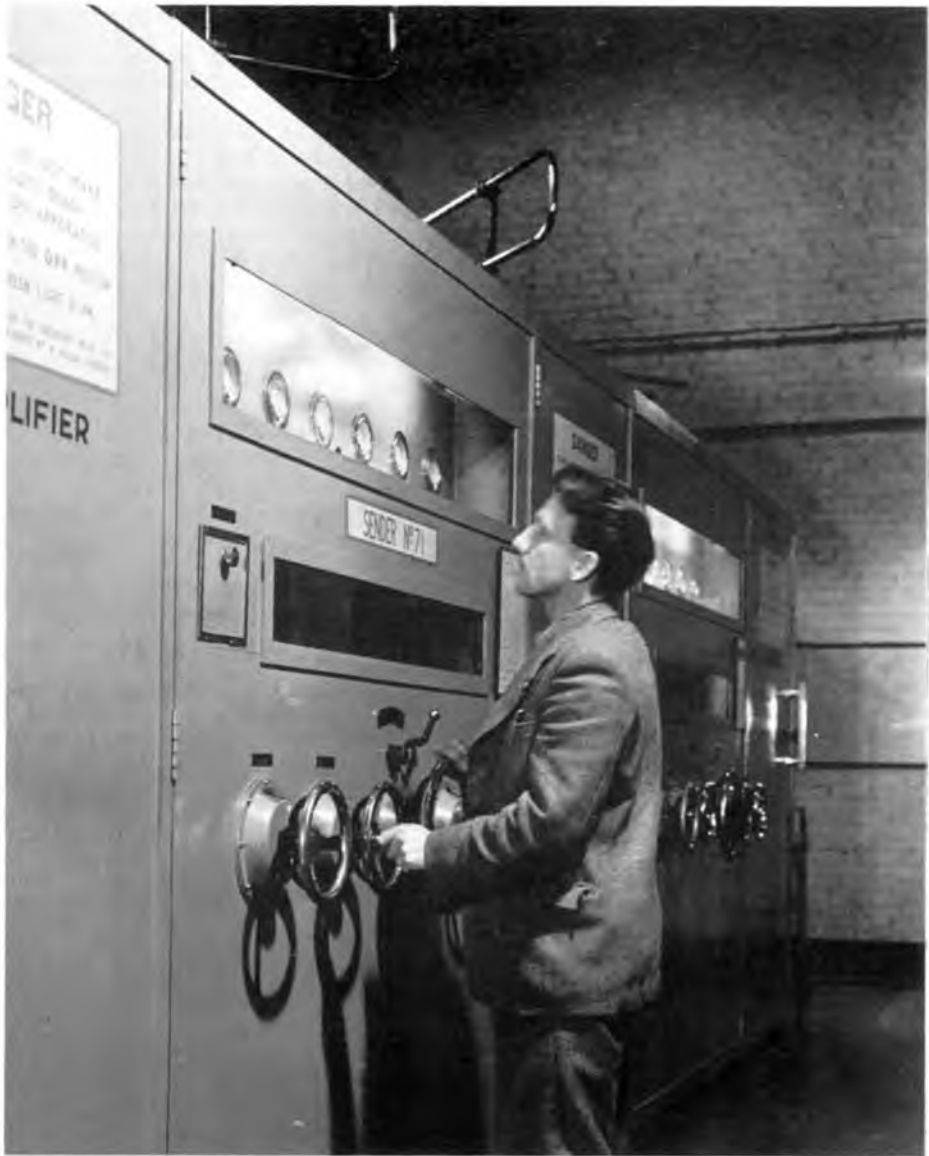
All transmitters on short wave were called "SENDERS", this picture shows one of the original Senders at SKELTON B ex. OSE 9 having some fine tuning on one of its two 100 kilowatt channels adjusted by a Technical Assistant in the early 1950s. This is one of the highly technical duties performed for over forty years by young men such as the one shown here who helped Skelton keep the nation in touch with the World.
