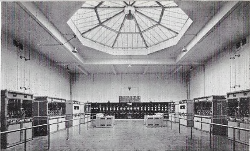
The transmitter hall at Westerglen
