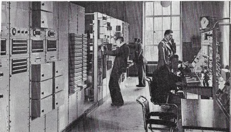
The control room at Broadcasting House, Glasgow
