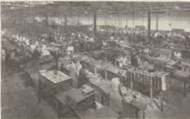
This is a general view of the final assembly and packing department—the last stage in G.E.C. battery making and a very important one, too
