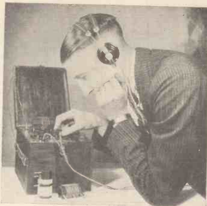
Adjusting the controls of the Midget short-waver, a sensitive little set that will bring in the whole world—on headphones, anyway. Note the extra plug-in coils
