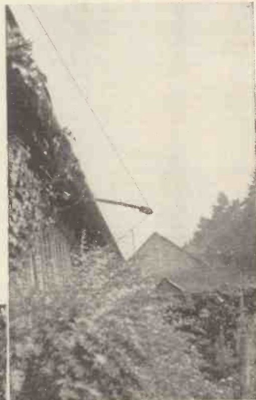
The lead-in arrangement. Note how a stand-off insulator keeps the wire well clear of the house
