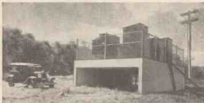
Part of the WABC transmitting plant, which is about 30 miles from New York
