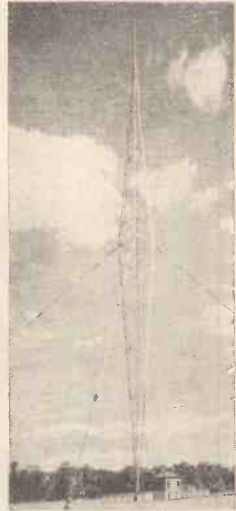
(Left).—Views of the top and bottom of the aerial mast at WABC. (Above).—The complete 600-ft. mast, shaped like an elongated diamond
