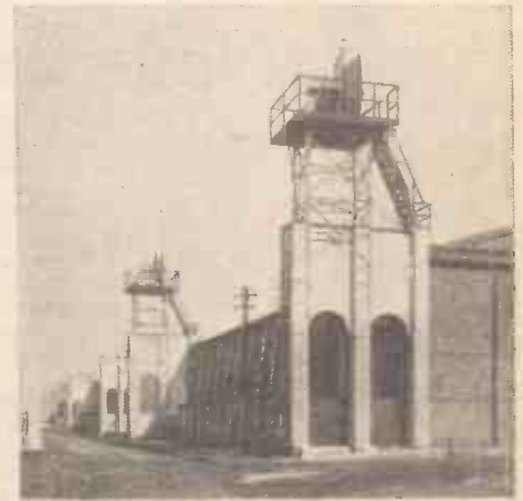
Aerials less than one inch long are used for the 17-centimetre signals, which are concentrated in 10-foot reflectors
