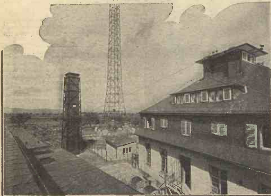
An unusual glimpse of the new Frankfurt station, which shows the base of one of the huge masts, the water-cooling tower for the valves and the elaborate lead-in arrangements. You can now hear Frankfurt on 259 metres with increased power
