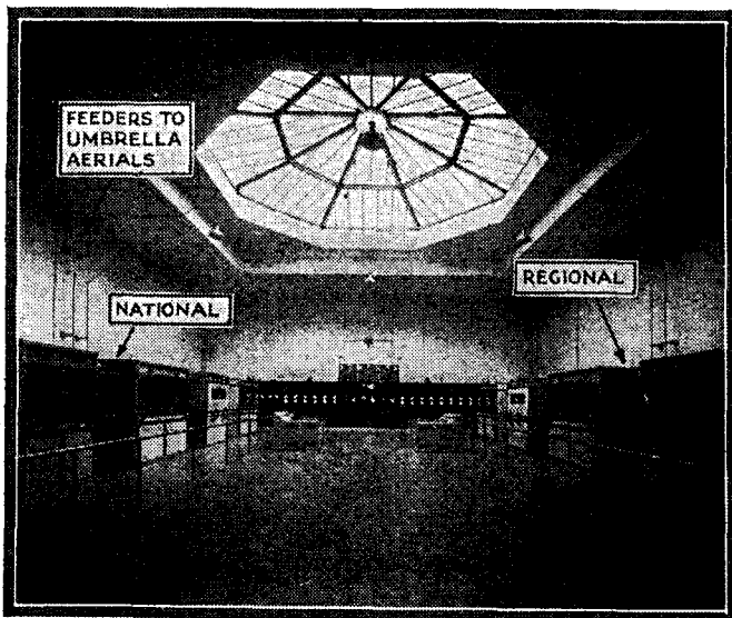
The transmitter hall at the new Scottish Regional station
