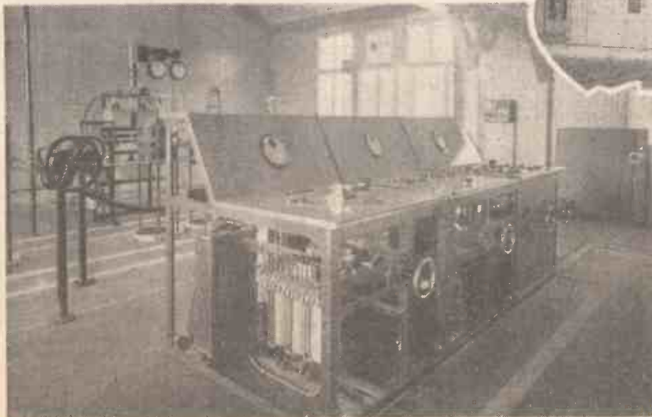
Two views of the newest of Yugoslavia's three broadcasters, Ljubljana, (oval) the station building and (left) the control desk at which the high-tension circuits are regulated. You can hear Ljubljana on 574 metres
