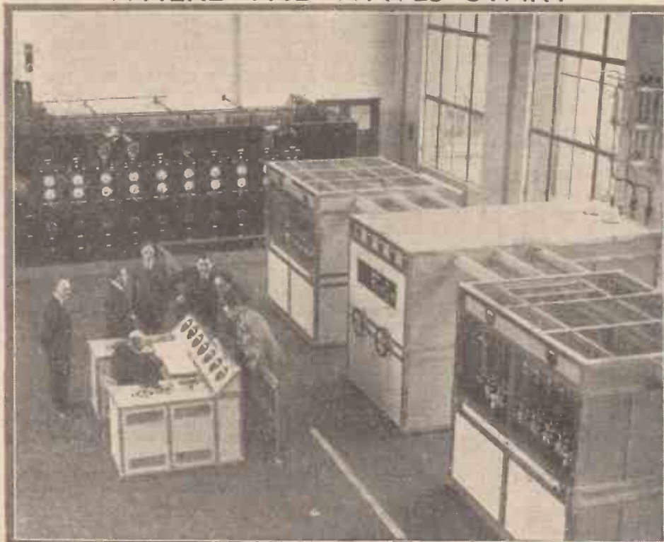
B. B.C. officials and some visitors discussing the North Regional Station inside the transmitter hall. One of the twin control desks is in the foreground, and the panels of one of the transmitters are at the right
