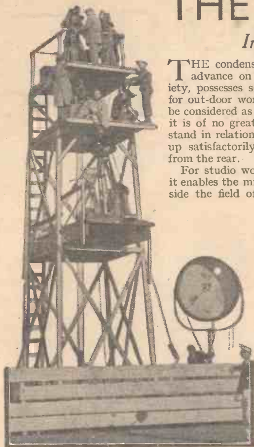
The beam microphone in use in a new talkie Cimarron : note the four cameras at different levels
