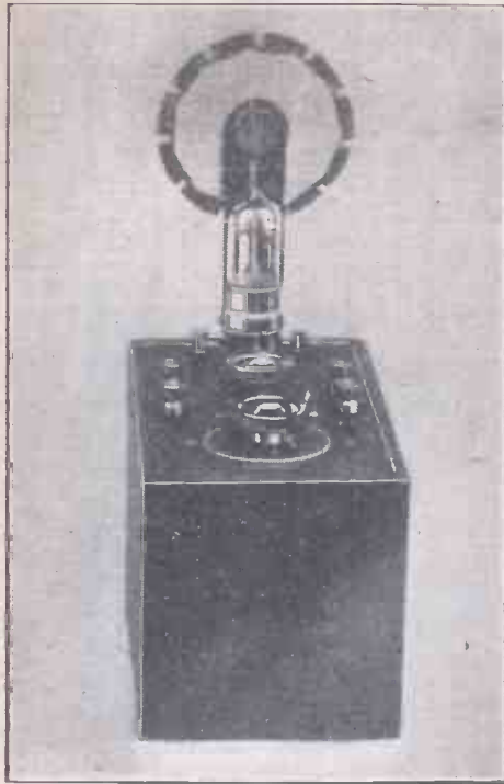
Fig. 4.—The Complete Wavemeter.
