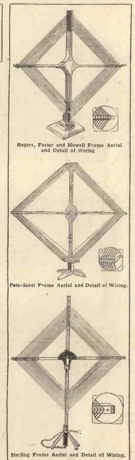
The length of wire used is 160 ft. This aerial turns in its socket, and can be held in position by means of the set-screw provided.
