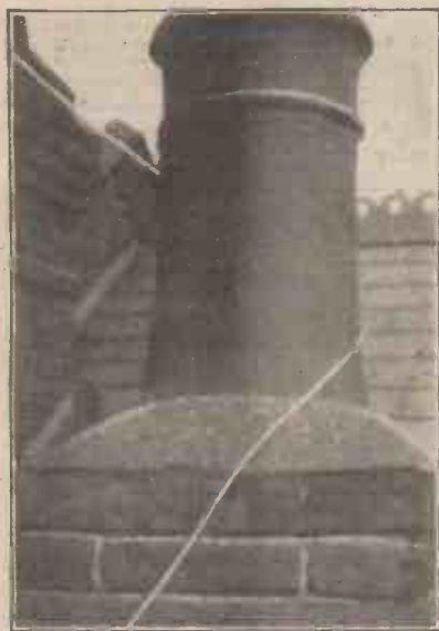
Photograph of Aerial on Chimney.
