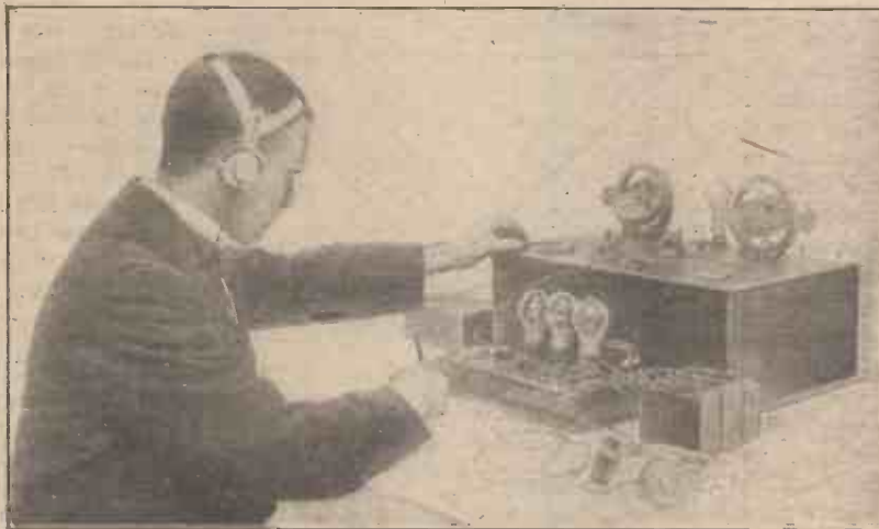
Operating a Four-valve Set.
