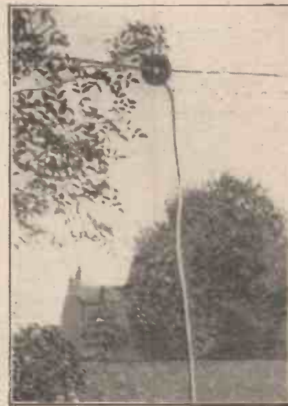
Photograph showing Down Lead and Adjusting Device.
