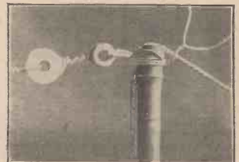
Fig. 3.—Photograph showing Wiring of Insulators and Spreader.
