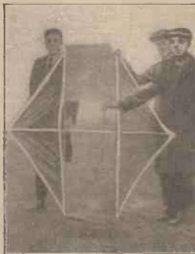
Fig. 2.—The Kite that Carried the Aerial.
