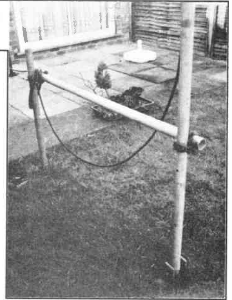
Photograph 3 Showing the mast locked in the desired direction with scaffold clamps
