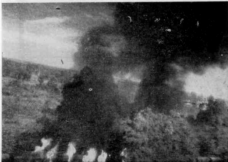
The result of a bomb-burst on a train carrying oil.
