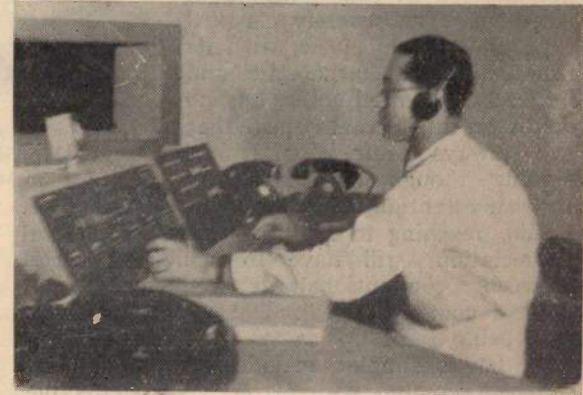
Control panels in the control room at the studio building, 8 Williams Road, from where the programmes originating in the various studios are controlled, amplified and then passed on to the transmitting station.
