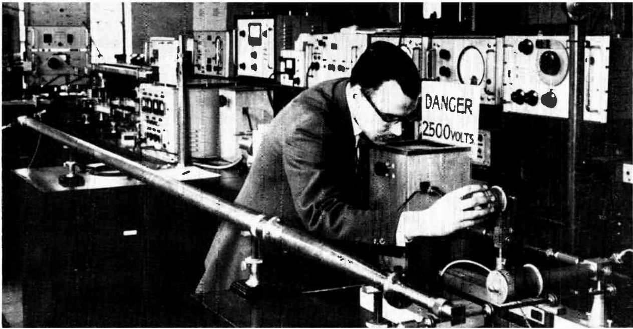
Millimetric waveguide research at the Post Office Research Station, London, England. The low-loss propagation of microwaves in cylindrical tubes over long distances has an enormous potential field of application in telecommunication.
