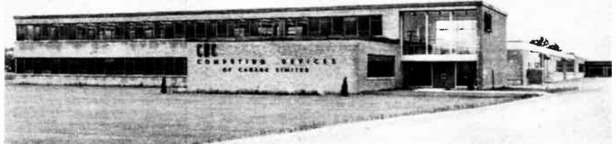
● The new head office and plant of Computing Devices of Canada Limited at Bell's Corners, near Ottawa, Ontario, provides 82,000 square feet of office, laboratory, and manufacturing space to accommodate the rapidly expanding activities of the company.
