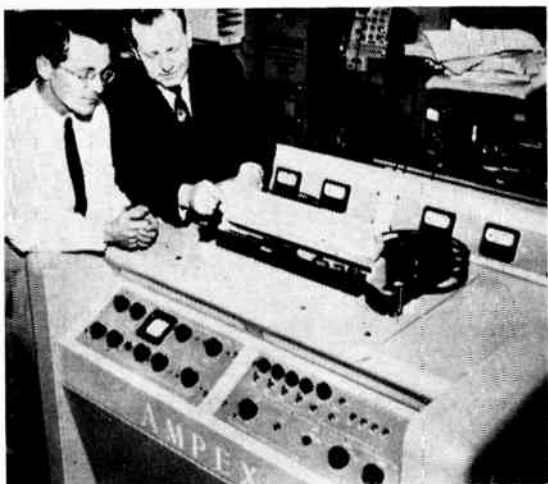
● Senior project engineer and Phillip L. Gundy, manager of the audio division, inspect the magnetic head assembly of the new television tape recorder.
