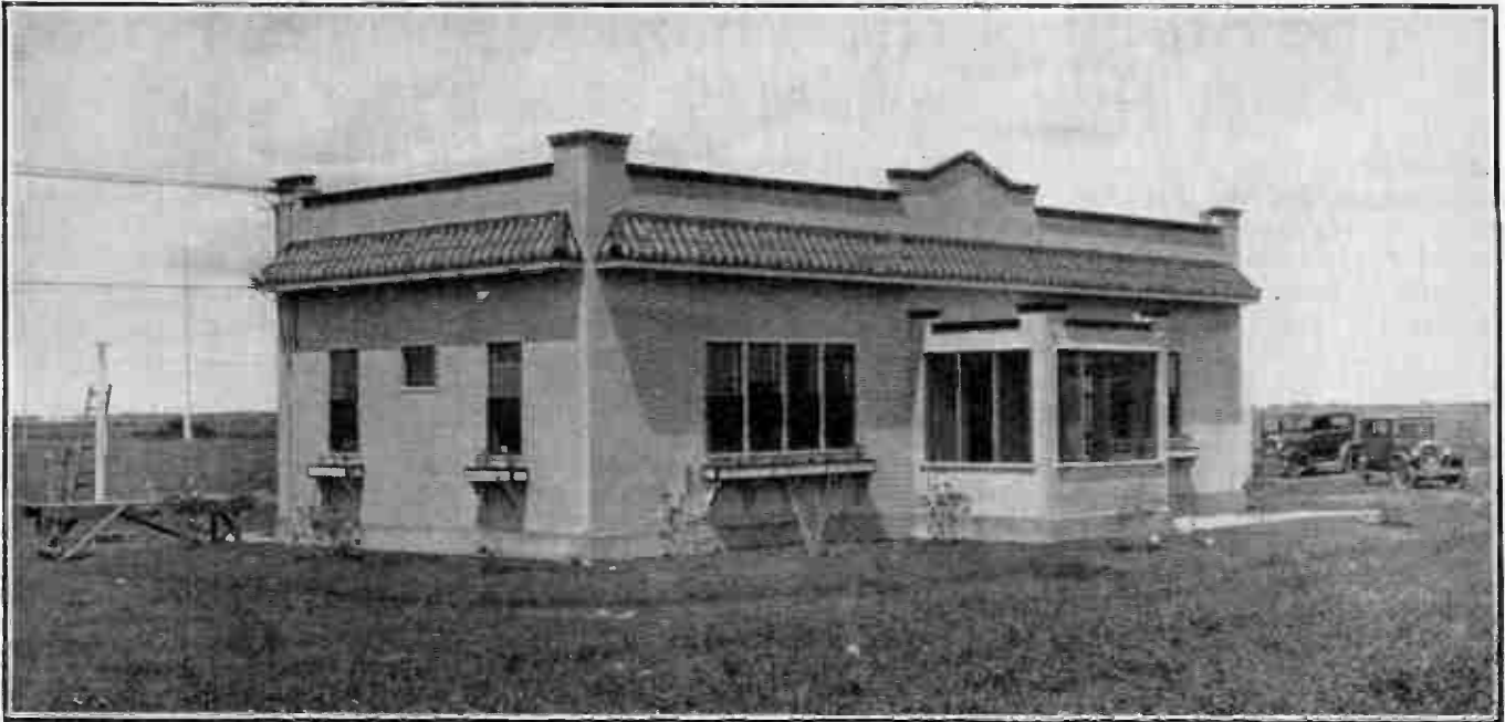
The Transmitter house of CJRX, a short-wave station at Winnipeg. It is located at Middle Church, a few miles north of Winnipeg. In the same building are a number of short-wave transmitters by means of which, on other wave-
