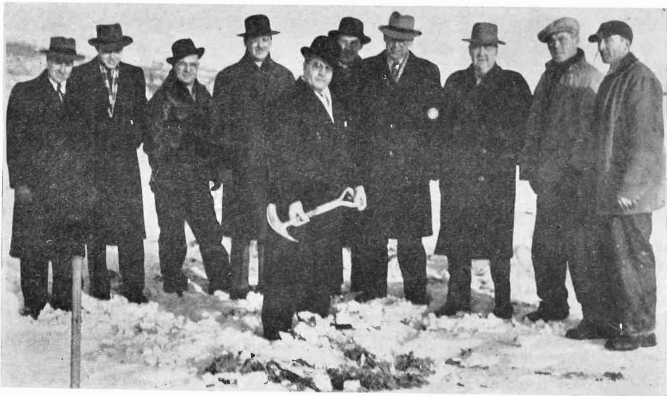
MAYOR BEATON OF SUDBURY, TURNING THE FIRST SOD
