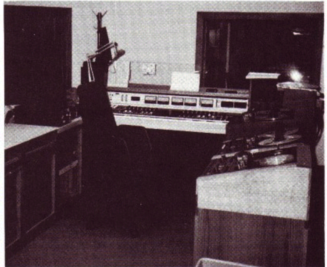
to the finished studios.
