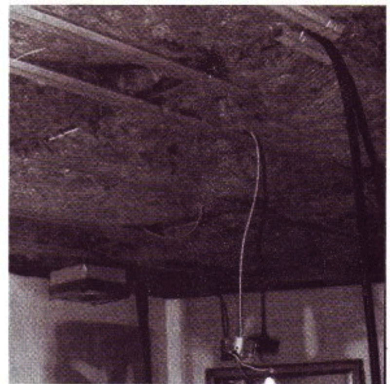
Ceiling sound blanket in place.
