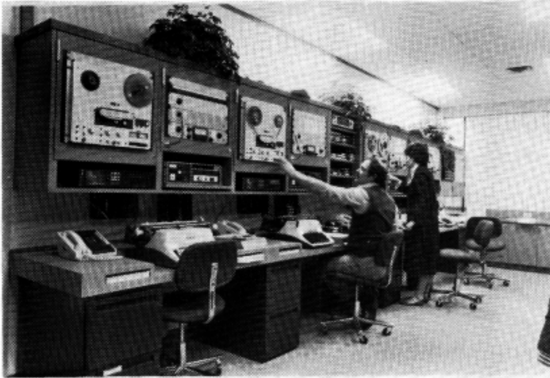
Newsroom has four work stations, each with a DTL switcher, Revox PR-99 tape machine, ITC cart machine and a Technics M280 cassette machine.
