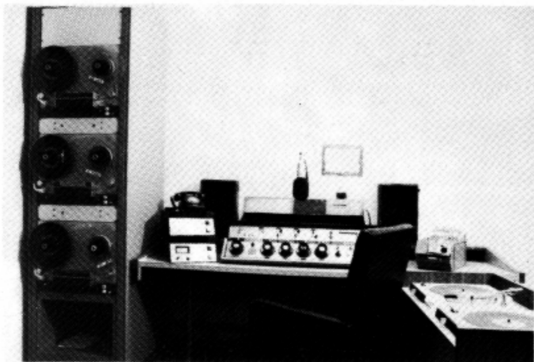
Emergency studio at transmitter building, with three tape machines at left.
