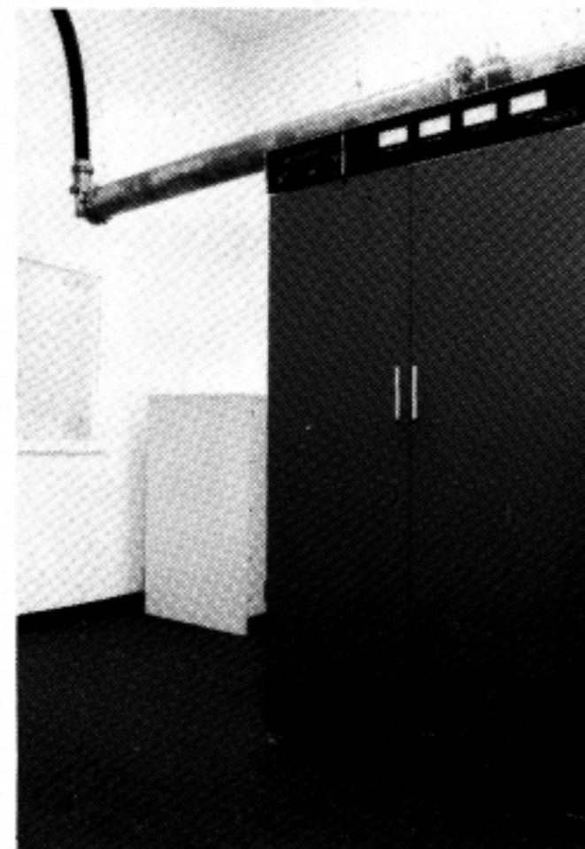
CKLA-FM transmitter [Harris FM20K]; 9 kV power supply is separate cabinet.
