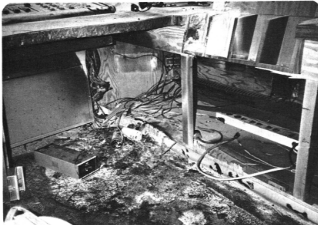
A view under the console where fire started.
