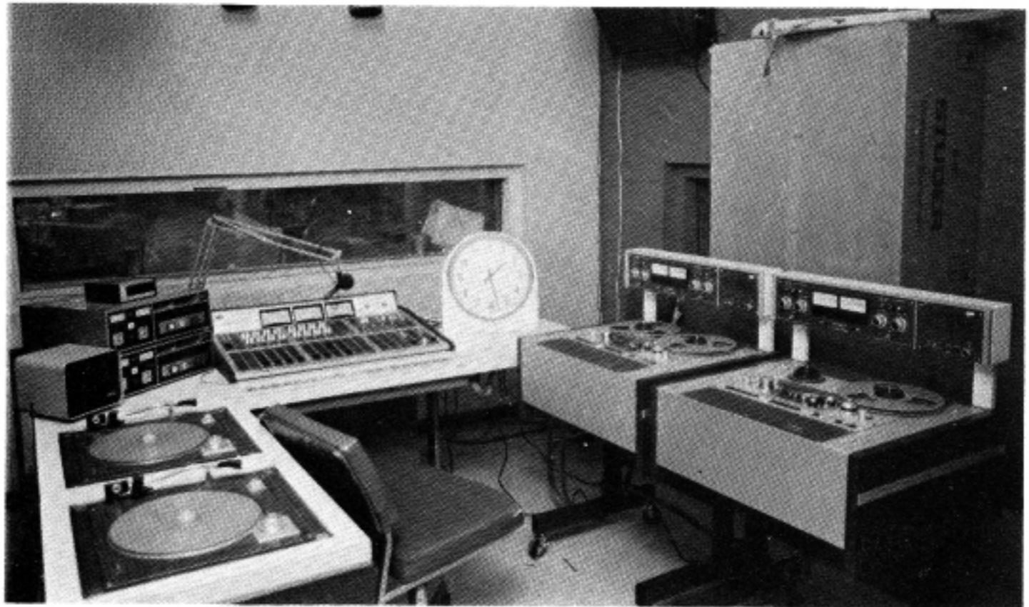
Master control room was added to Fanshawe's four existing studios in Radio Broadcasting course. Equipment includes McCurdy 7550 console, Technics turntables, Studer and Ampex reel-to-reel recorders. ITC cartridge machines are used throughout the radio and journalism studios.
