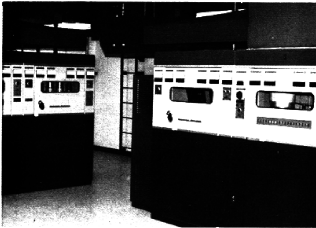
New 50 kw Contintal transmitter at CKOC Hamilton.
