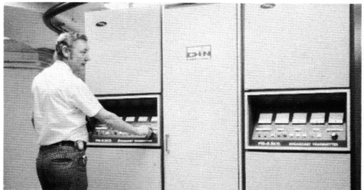
Paul Hunter, vice-president and director of engineering at CHIN-FM adjusts station's AEL transmitters located at the 1200-foot level of Toronto's CN Tower.
