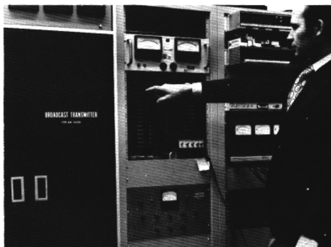
Station engineer Ray McMurray checks out CCA 1kw standby, part of all-new transmitter plant.
