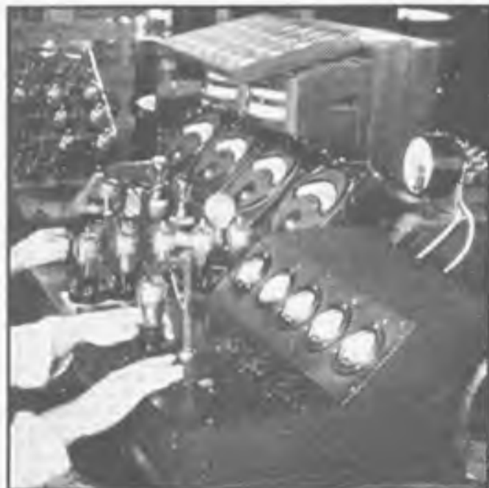
Electrical Inspection Tests
