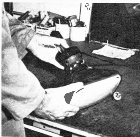
The easiest way to test for a bad picture tube is to install a test picture tube in its place.
