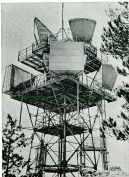
FIG. 1-26. A radio relay tower used for the reception and transmission of television signals.
